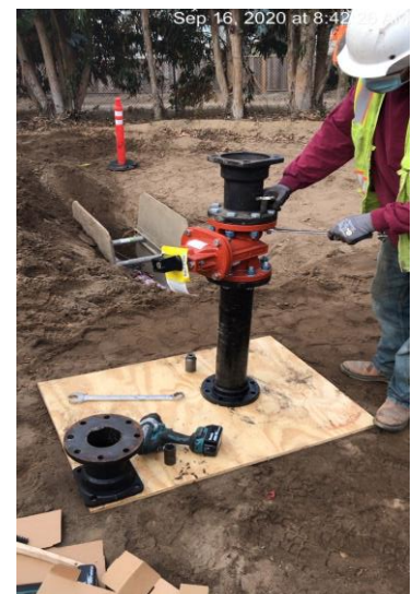
Valve assembly for blow-off
