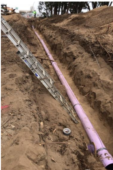
Recycled water pipeline
