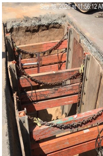
Shoring for pipe receiving pit
